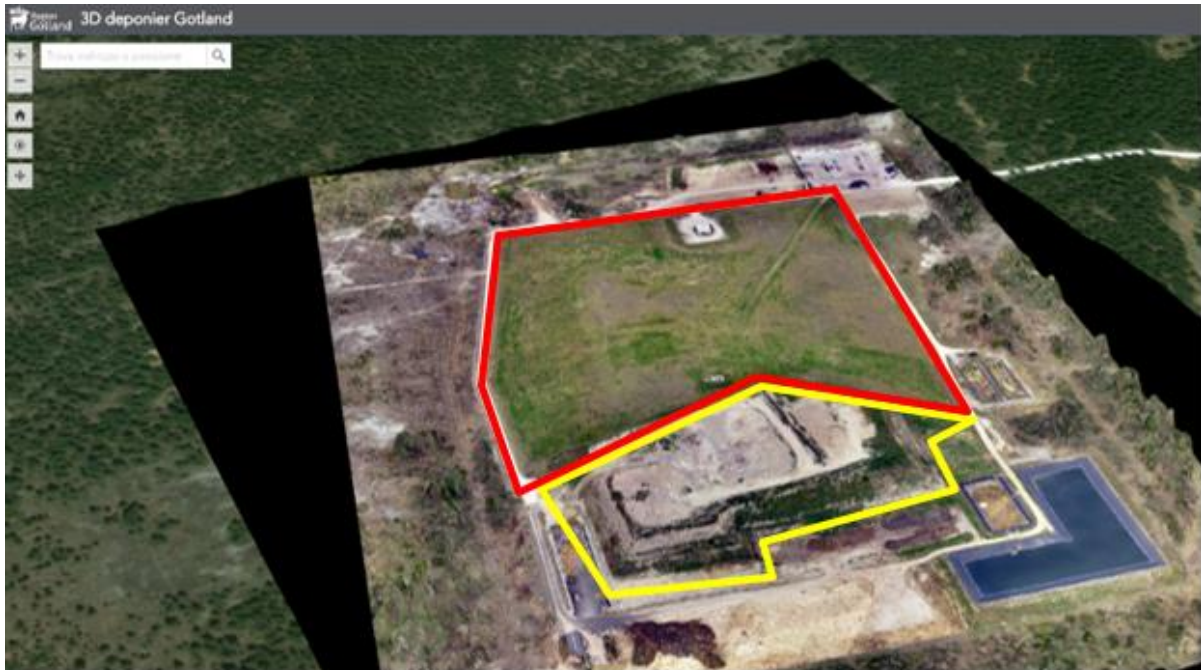
Figure 2.2 The areas delimited by yellow and red lines represent active and closed parts, respectively. In the upper right corner, there is a recycling station. On the right side of the landfill, the leachate treatment is located. South of the landfill, there area composting areas. Aerial photo from ReSource/Region Gotland.
