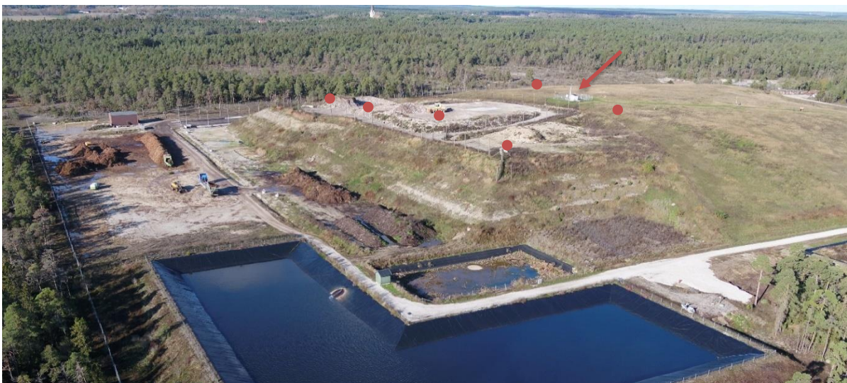
Figure 2.1 Overview of Slite landfill site. The flare at the top of the landfill is shown by an red arrow while gas collection wells are marked with red dots. The composting pile and garden waste are shown in the figure. Aerial photo from ReSource/Region Gotland.
